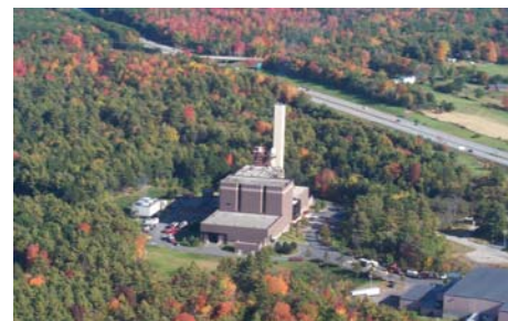
Figure 5: ecomaine WTE, Portland, Maine
