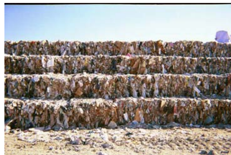
Figure 7: An example of a balefill [5]
